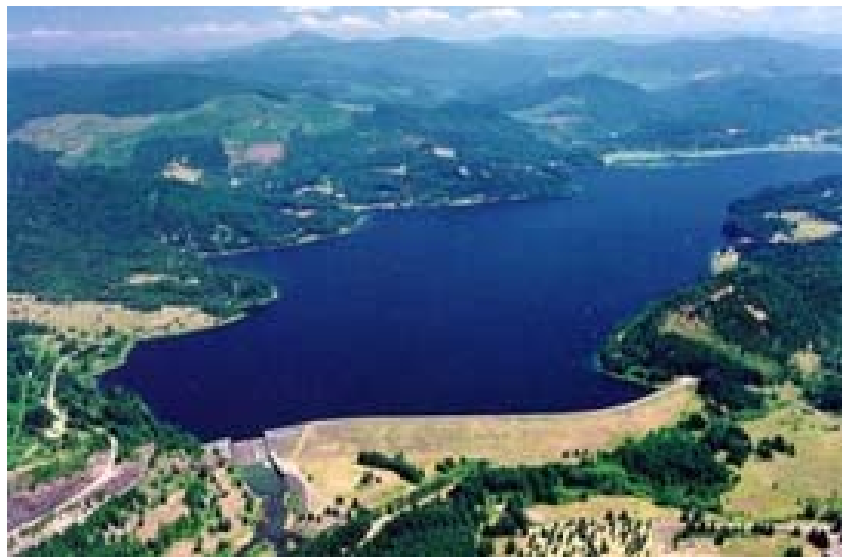
Figure 2.1 - 2 - Photo of Dorena Lake Dam
